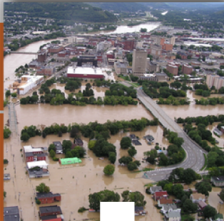
2011- Flood, the YWCA was evacuated for several days and luckily only had to replace the boilers and one water heater due to damage.
